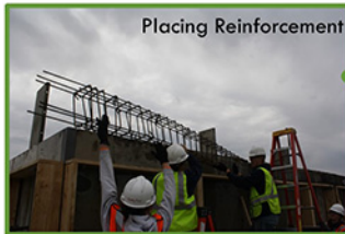
Reinforcement Preparation
