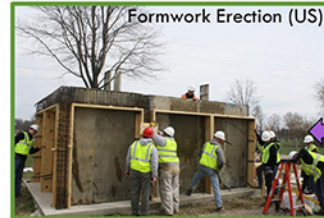
Formwork Erection (US)
