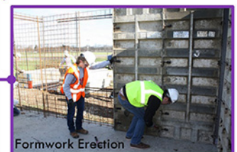
Formwork Erection
