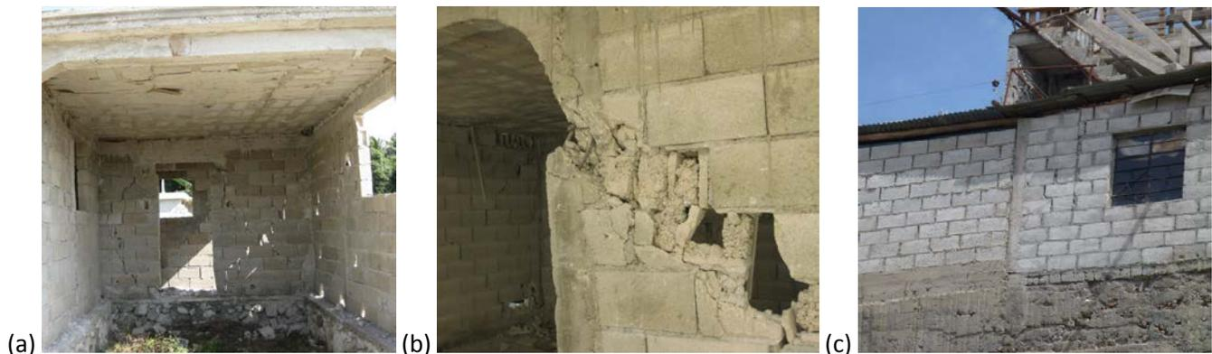
Fig. 1. Typical home in Léogâne, Haiti, (a) built with CMU (concrete masonry unit) walls and undersized columns (note shear failure in wall in the background); (b) shear failure of CMU wall transferred forces into neighboring column; (c) compared to typical CMU home in Quito, Ecuador, having same construction modality as home in Haiti. Note the complete absence of beams in both homes.
