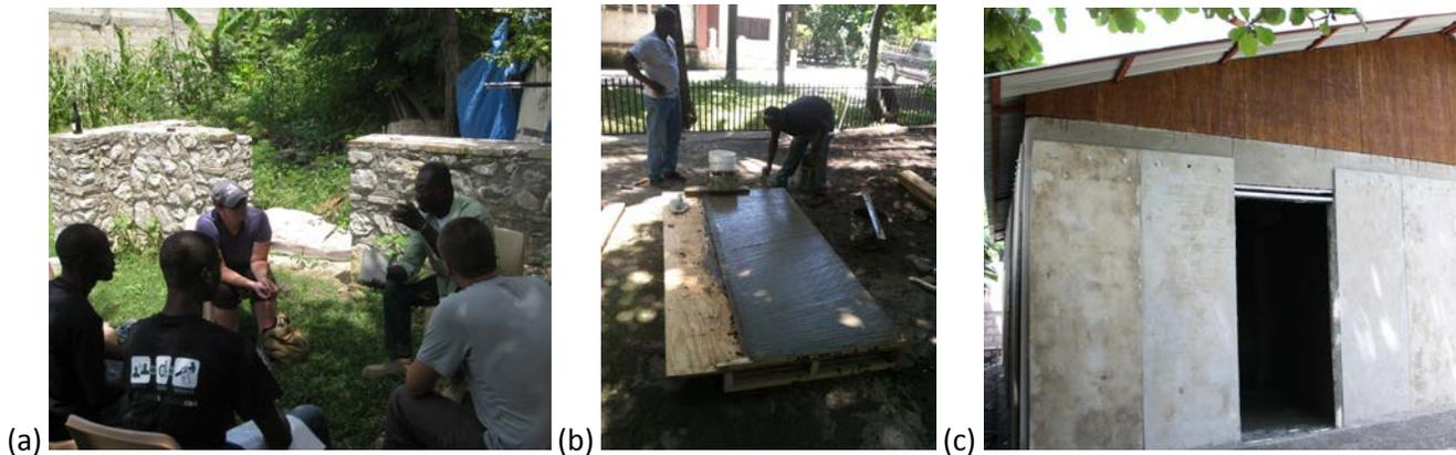
Fig. 4. (a) Discussion with Haitian architects during the solution incubation process; (b) concrete panel production in Haiti and (c) structure built with concrete frame and panel system.
